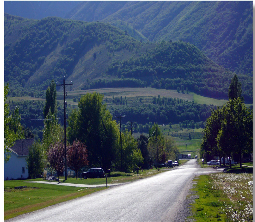
Traditional local residential streets have pavement 22 feet wide with no curb and a drainage swale that is kept green and maintained by adjacent property owners.
